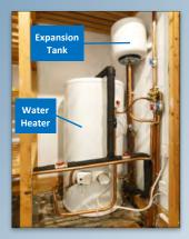
overflows from the main hot water tank and pushes against an air cushion within the expansion tank, causing the air cushion to compress and allowing water to flow in. This alleviates the pressure of thermal expansion by giving the expanded hot water a place to go. The size of the expansion tank depends on the size of your hot water tank, the water pressure, and water temperature.
